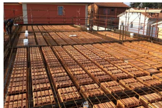
Solai in laterocemento
