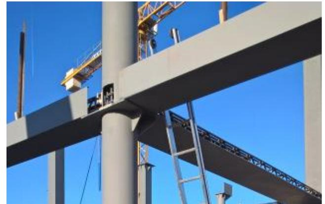
*PREM System – composite steel-concrete technology*
