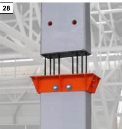
It is a temporary steel shelf placed on bushings, with nuts and washers, able to support the first phase loads until the completed concrete is cast. Then it can be easily be removed and reused. The advantage of this typology is not to have, at the end of the construction, any encumbrance to the beams intrados, just like with the solution without shelves with the advantage of not having to taper the bars, but the disadvantage lies in its greater cost.
