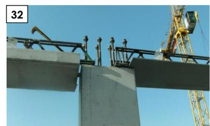
*Fig. 30, 31, 32 – reinforced concrete and composite steel–reinforced concrete PREM beams on wet structural joint prefabricated columns without shelves*
