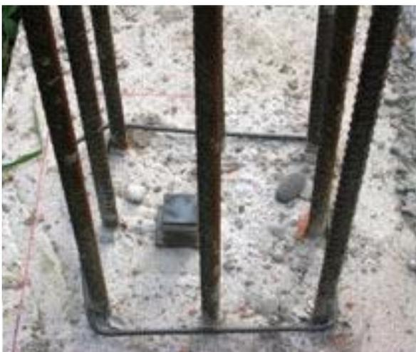
Inside the bars previously embedded by the contractor, a stack of small size steel plates is placed in a central position, so the floor shelves are at the correct level. The plate fulfills the fundamental function of keeping the column raised from the foundation to allow its connection by means of the mortar. The assembly maneuver shown here is the same even in the case that the bars come out of the column intrados and the corrugated sheaths are positioned in the foundation.
