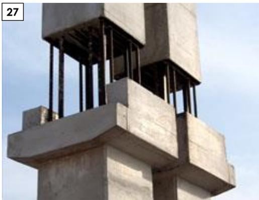
This solution supports both the first and second phase loads thanks to the larger dimensions and appropriate reinforcements set up into the shelves. The integrating reinforcements of the beams converge to the joint, and the complete castings is made only to guarantee the monolithism for the transmission of the moments to the column and the other beams converging into the joint. Less aesthetic appeal and production costs are evident.
