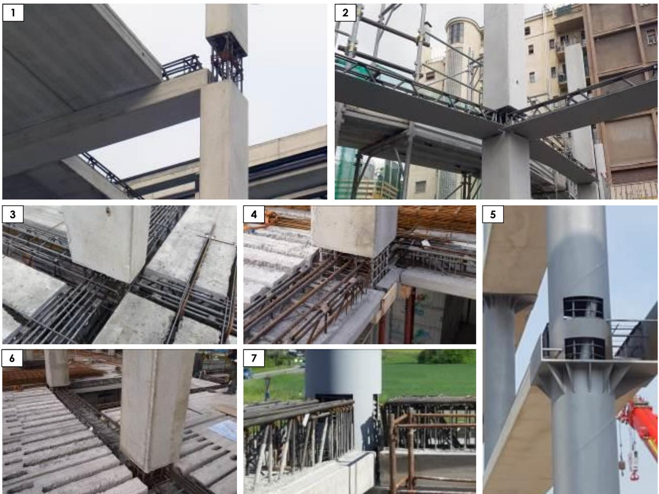
*Fig. 1, 2, 3, 4, 5, 6, 7 – Wet structural joints typical of PREM Building System*
