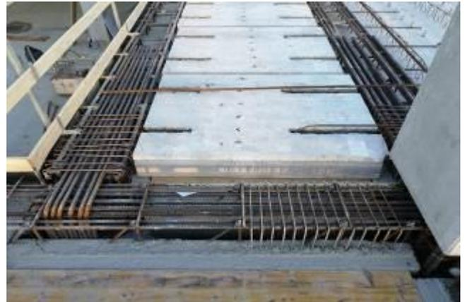
*PREM System – reinforced concrete technology*
