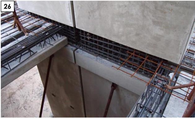
This solution provides sufficient bearing capacity only for the first phase loads, while the second phase loads will be transmitted directly to the columns core through the integrating bars of the beams and the concrete.
