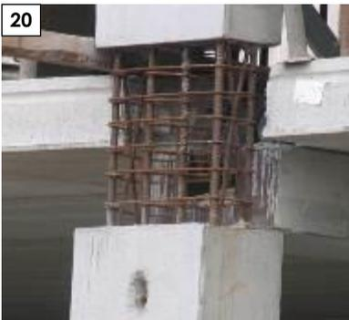
In order to guarantee a proper support to the beams in the casting phase, a more compact column reinforcement cage is formed, which is overlaid to the lower and upper cage and appropriately sized to consider the reduced geometry and supply the due resistance during laying phase. The solution presents the maximum appeal against higher costs of reinforcement and laying, and a greater accuracy both in the design and in production phases.
