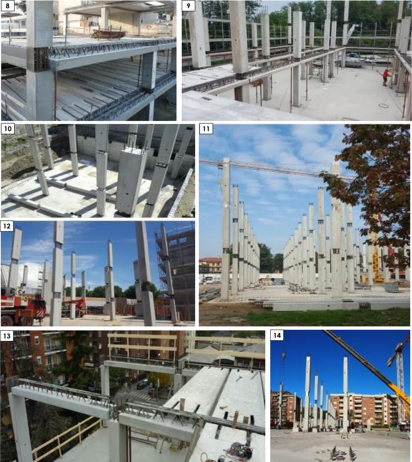
Fig. 8,9,10,11,12,13,14 – Typical images of prefabricated wet structural joint columns
