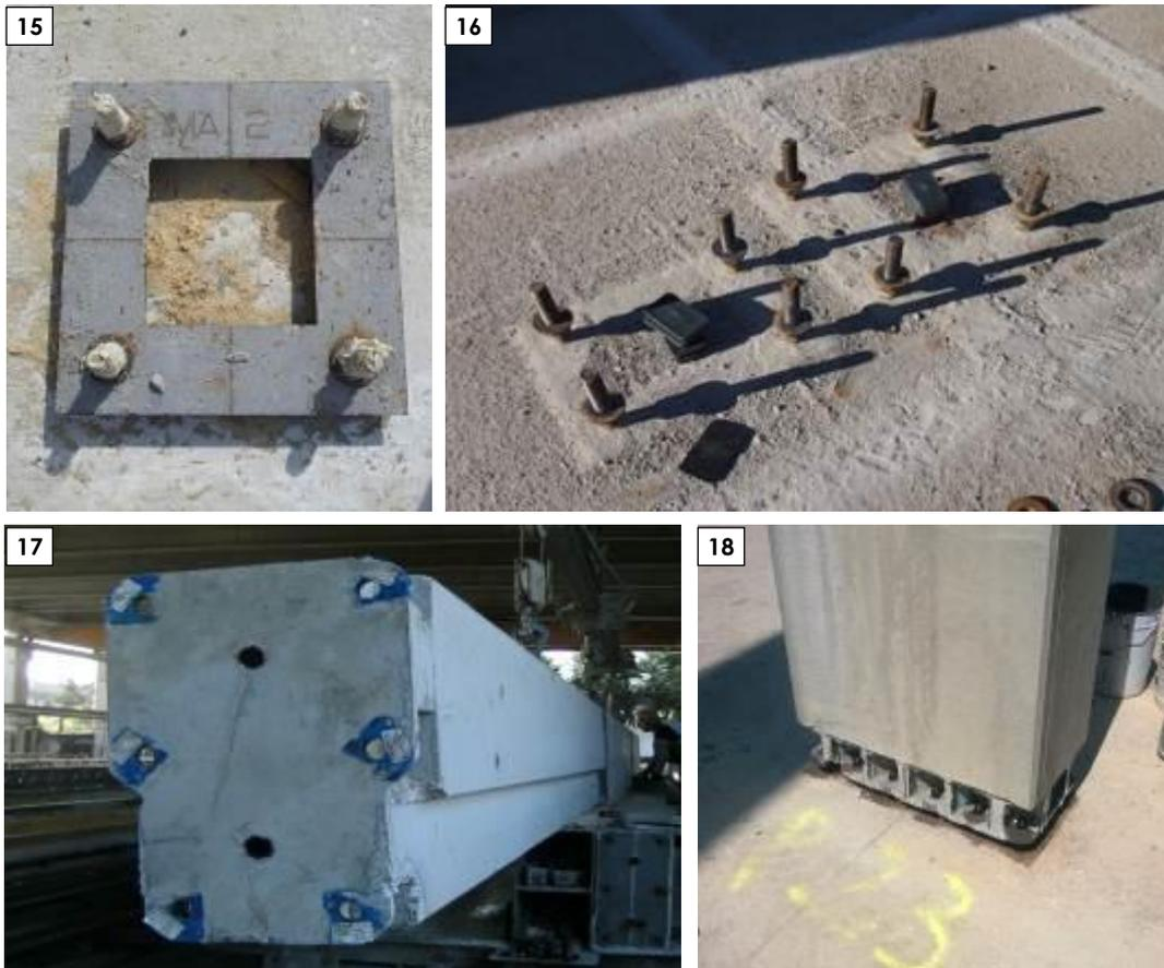
Fig. 15, 16, 17,18 – Connection to the foundation with prefabricated "shoe".
