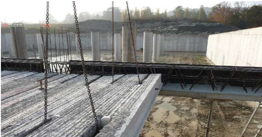
Azienda Agricola (BS): Travi PREM a2 – Solai a Lastre alveolari – Pilastri in c.a. in opera.
